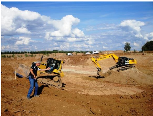
PHOTO No. 7 also shows Arne supervising
