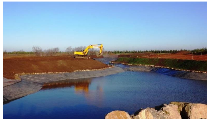
PHOTO No. 8 shows the completed irrigation lake
