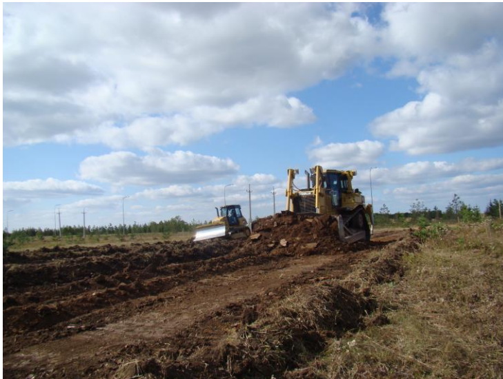
PHOTO No. 4 STRIPPING TOPSOIL
